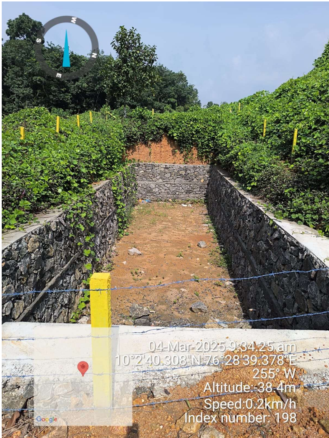
Drain and siltation pond
