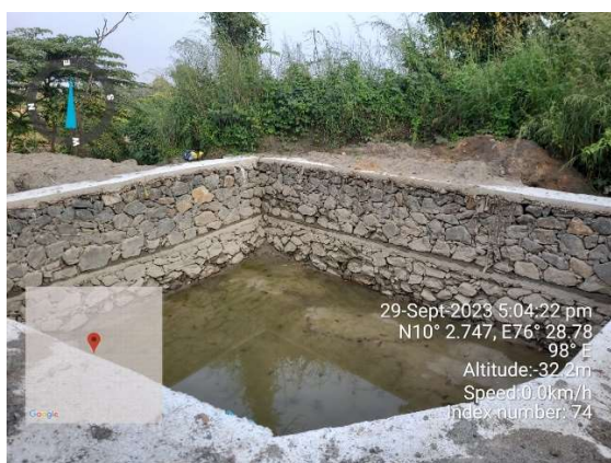
Drainages and siltation trap
