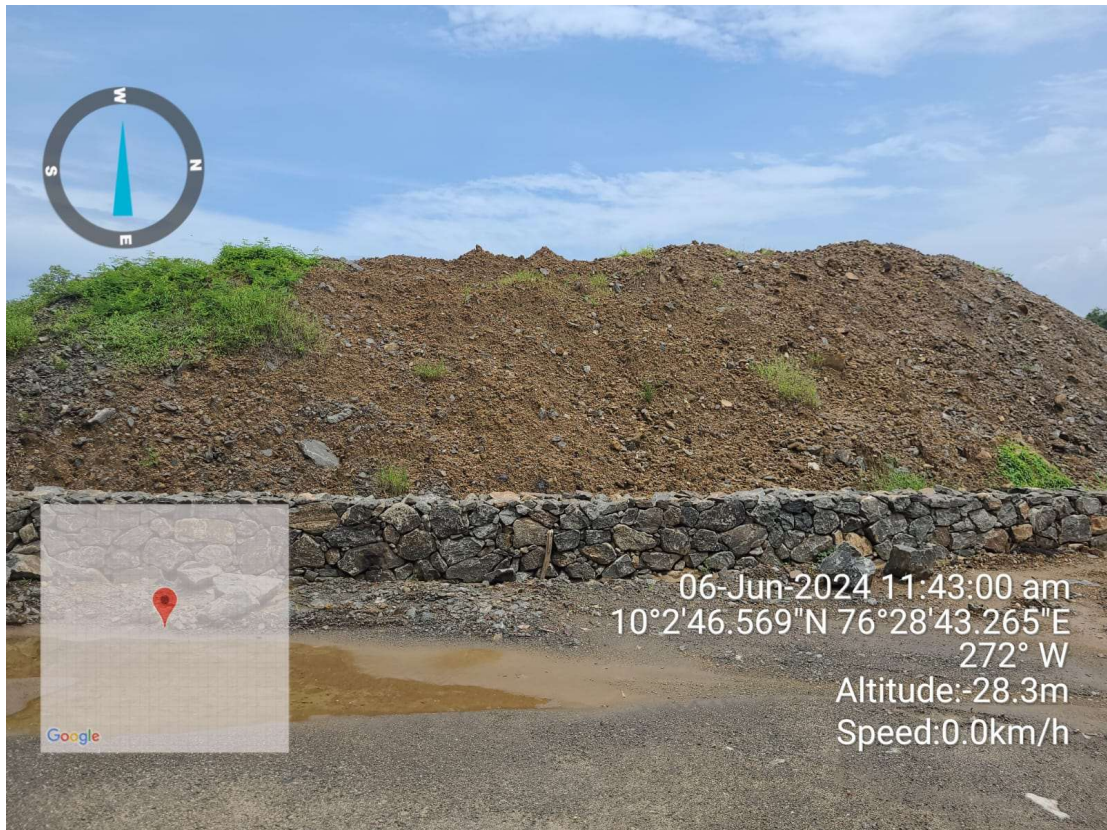
Dumping area with Retaining wall
