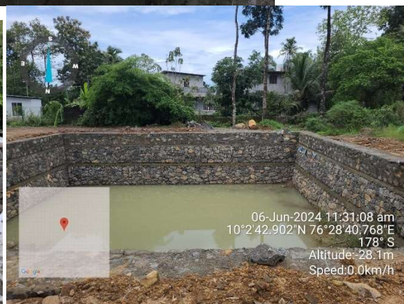
Drainages and siltation trap
