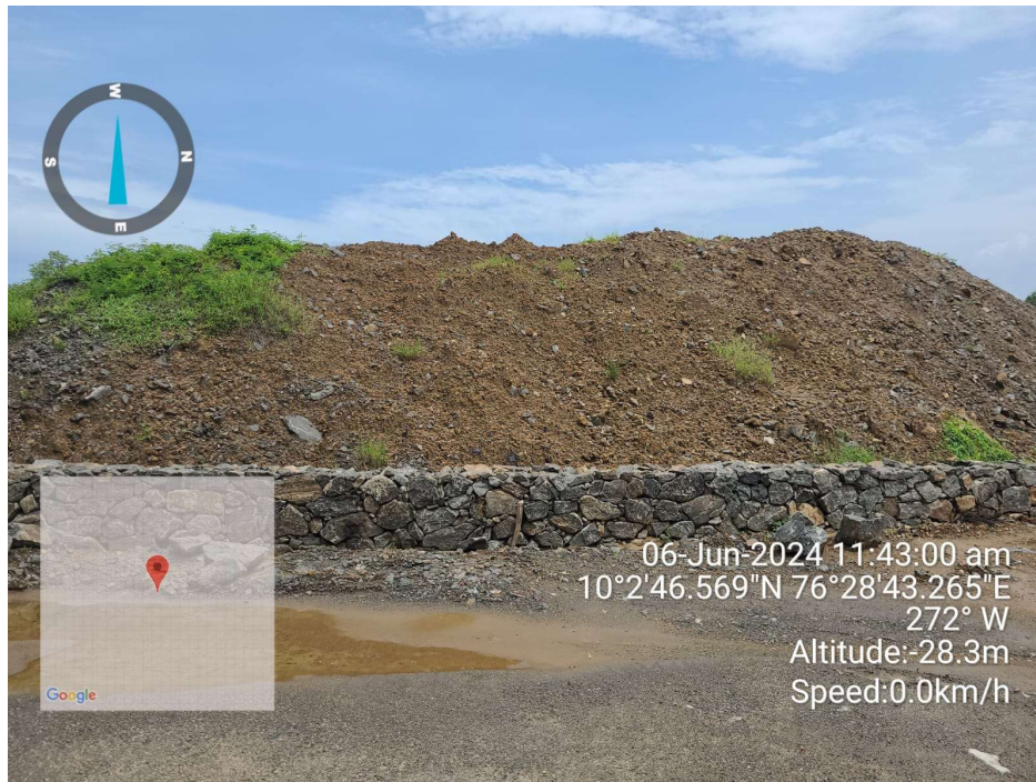
Dumping area with Retaining wall
