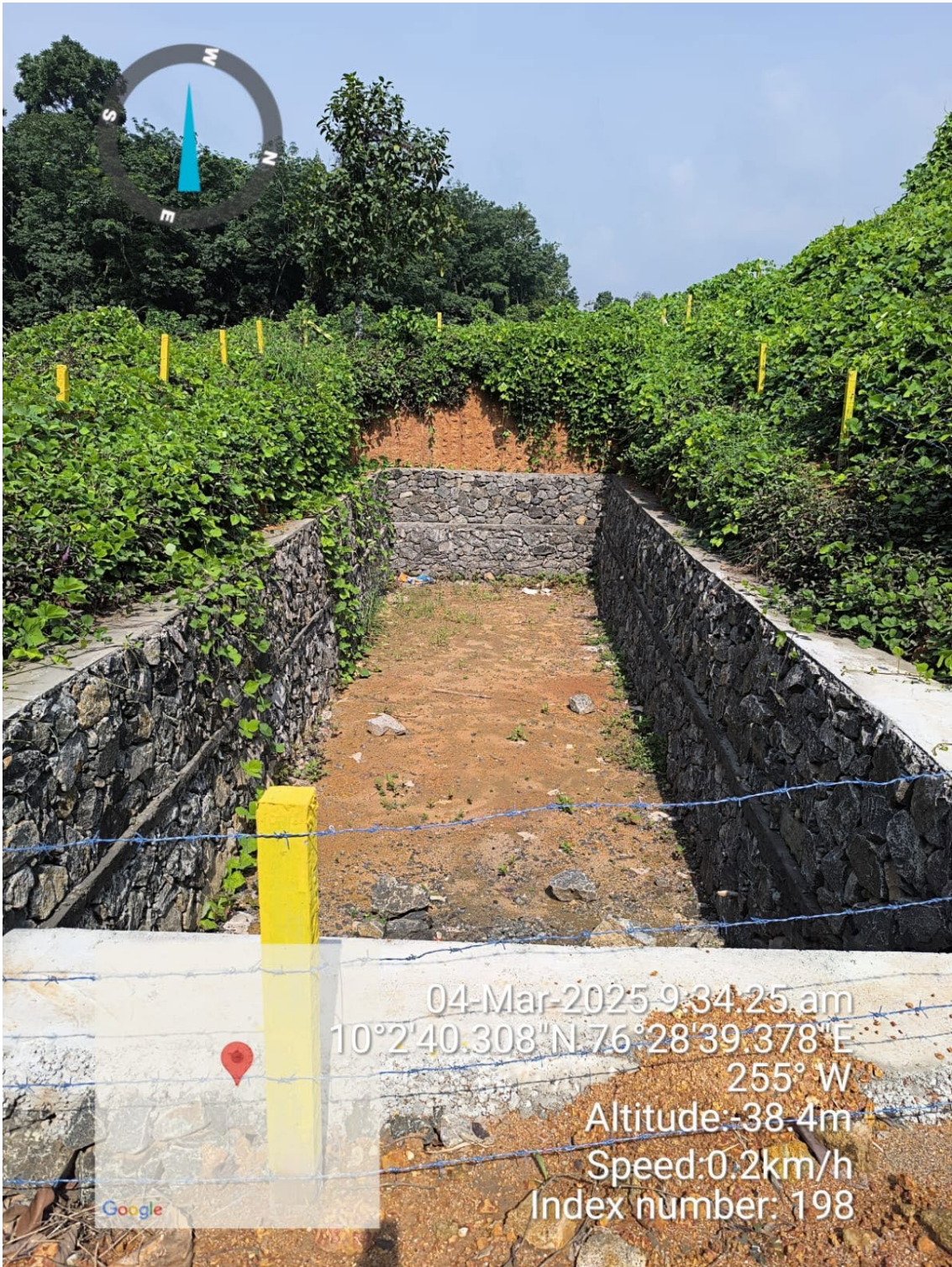
Drain and siltation pond
