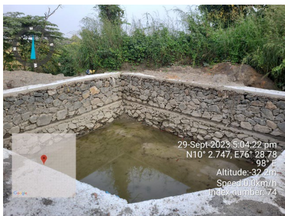
Drainages and siltation trap
