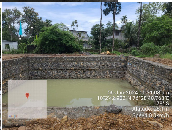
Drainages and siltation trap
