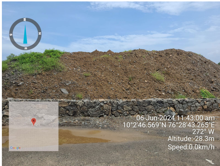
Dumping area with Retaining wall
